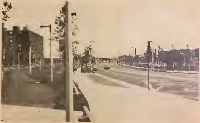
View of new Melnea Cass Boulevard approaching Washington Street.
